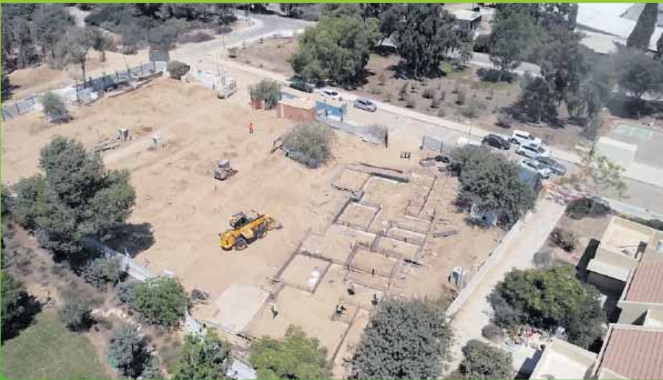
Early stage construction of new homes at Nir Oz.
